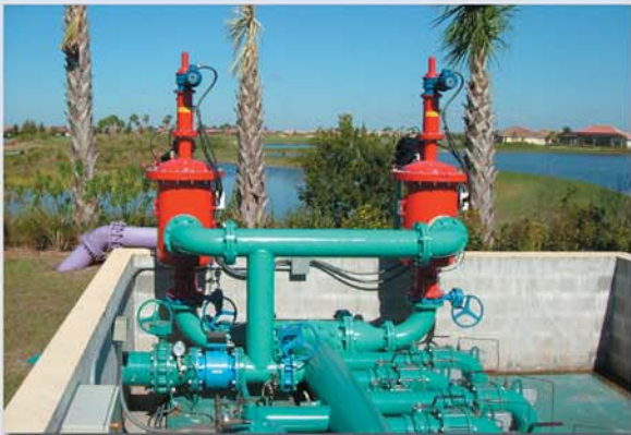
▲ Irrigation golf. 700m 3 /h, 200 microns. Tampa, USA
